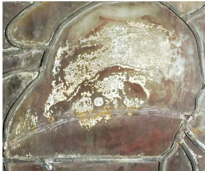
Corrosion of glass and paint surface due to moisture
